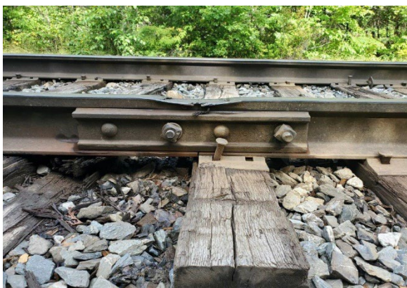
Figure 3. EMR track showing a deteriorated rail joint
